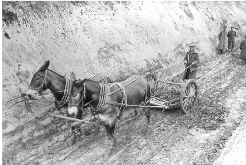
Grading for light railway construction.
